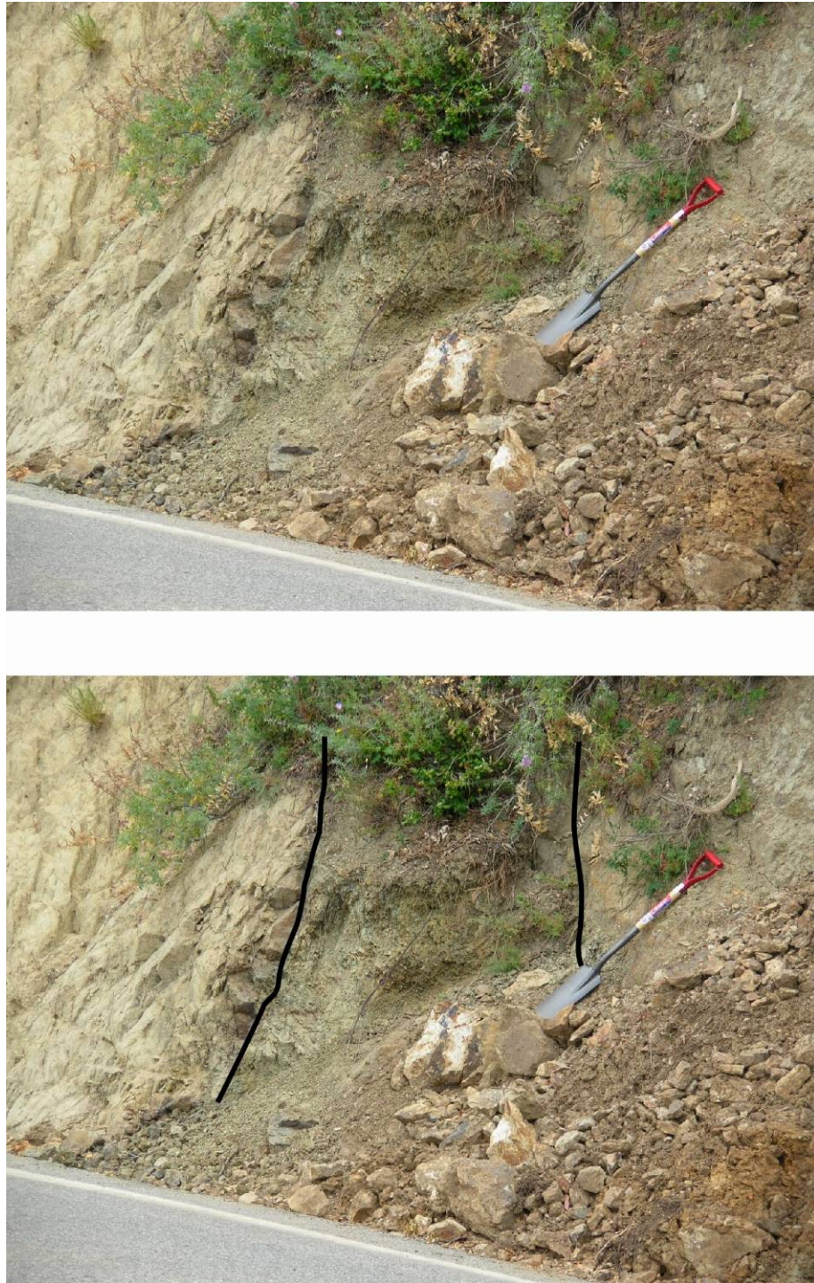
FIGURE 19. Fault at site C, an uninterpreted photograph at top. The same photo below with fault interpretation. Black lines indicate the edge of the fault zone. Note shovel for scale.
