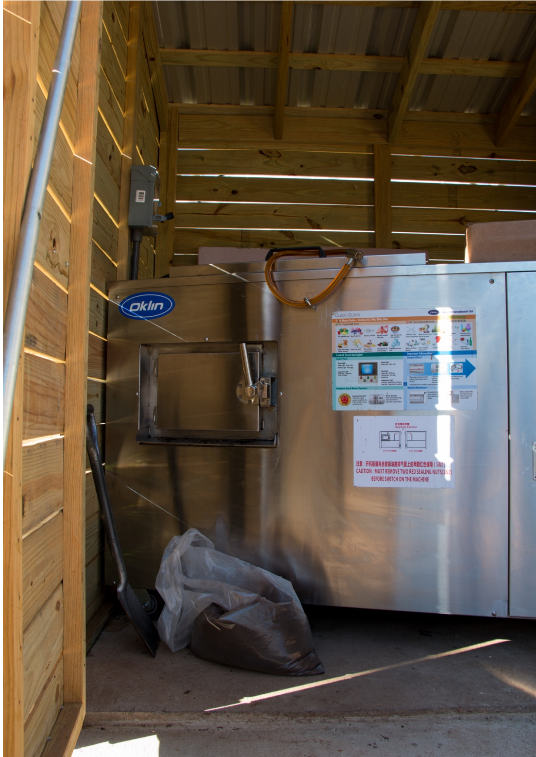
Figure 24: The Urban REAP composting machine turns compost into natural fertilizer for the garden at the facility as well as for purchase for people in Waco.
