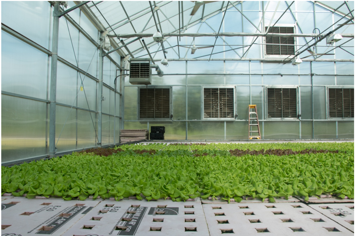
Figure 8: Ventilators at the end of the greenhouse along with fans suspended inside help keep the air fresh to promote lettuce growth.
