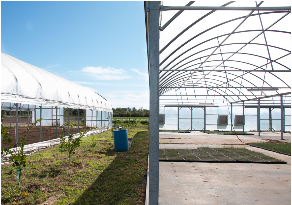
Figure 40: The greenhouses have retractable plastic walls that can be lifted for ventilation when the outside weather is optimal for seedling growth.
