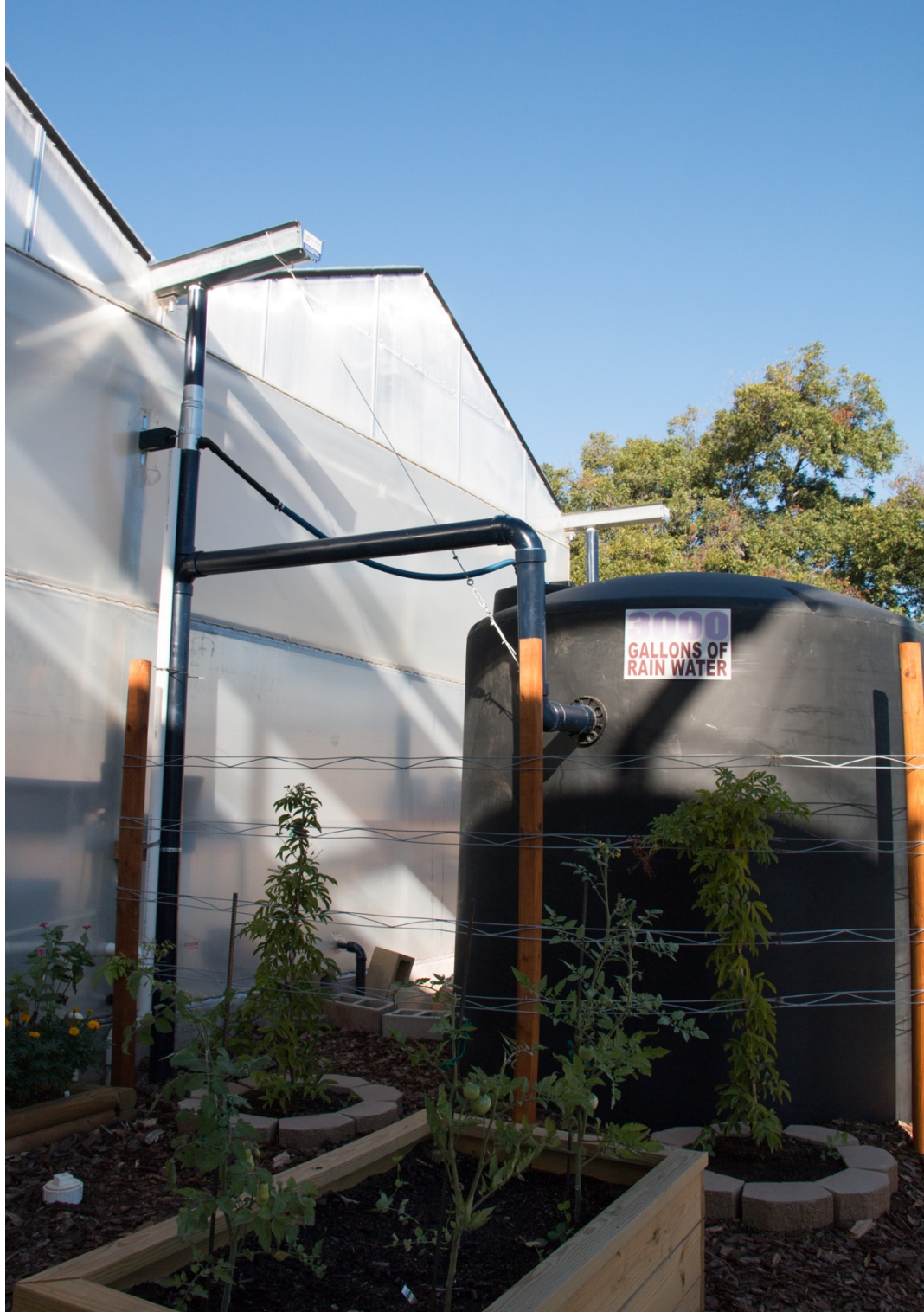
Figure 21: Rainwater is harvested through a gutter system on the greenhouse and is used as replacement water for the aquaponics system.
