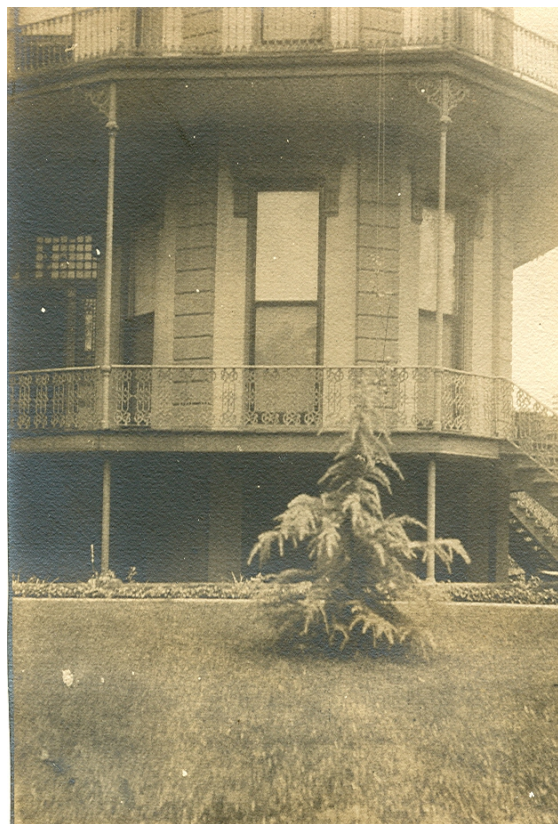
Figure 14. West porch and entryway, c. 1905. This photograph shows the cast-iron porch added to the structure's west side. Notice the difference in the railings on the first and second levels and the decorative brackets at the top of the small columns. On the left side of the photograph, the west door changed during the 1901 renovation is visible. Courtesy Texarkana Museums System.
